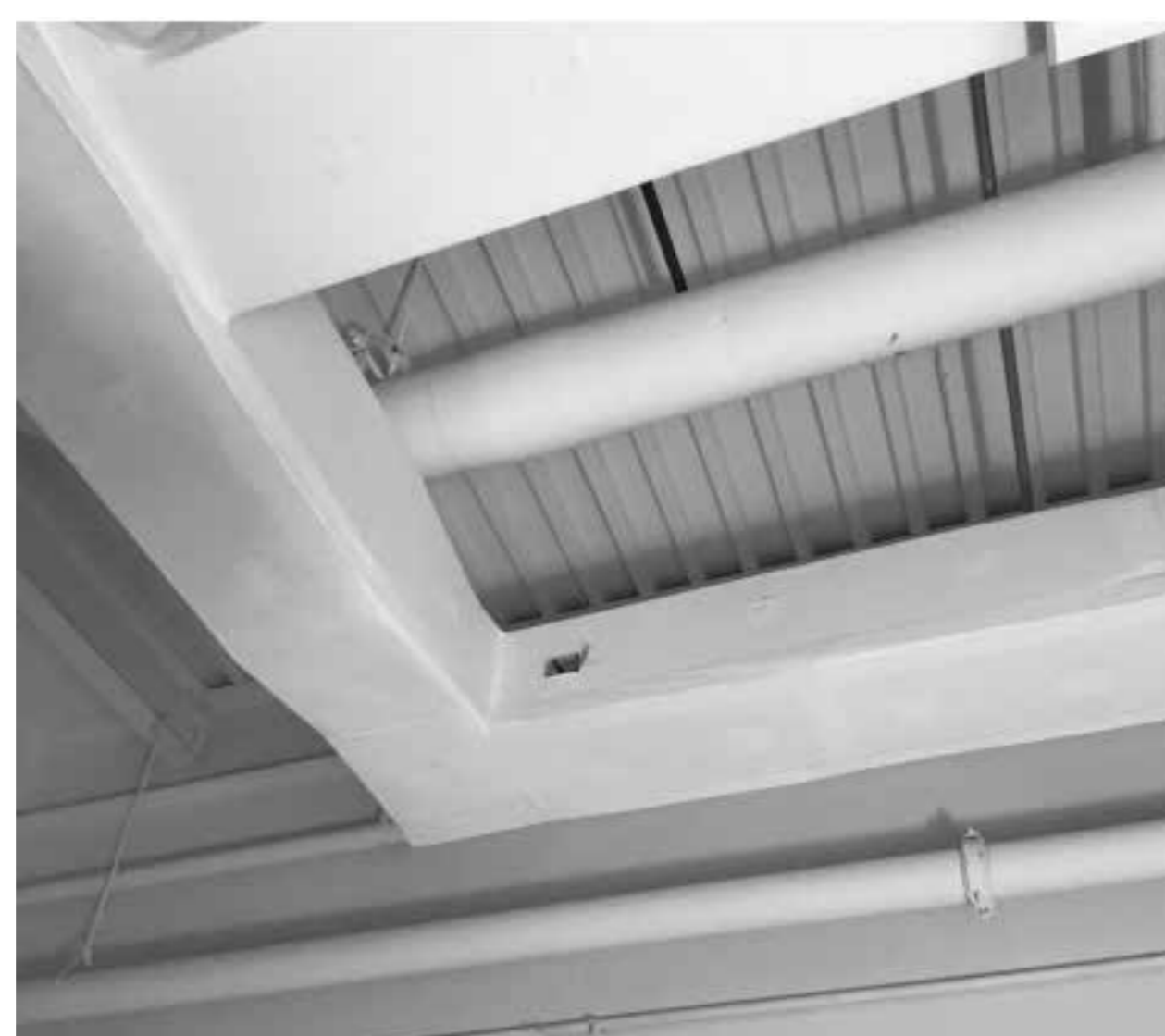
TYPICAL EXPOSED MAKE-UP-AIR RECTANGULAR DUCT
